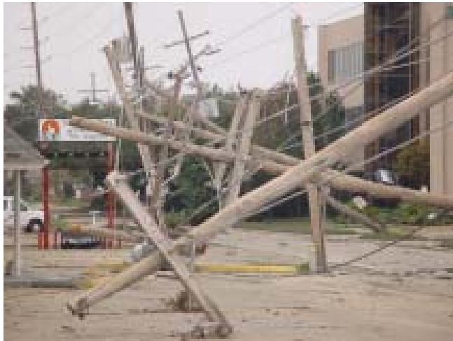
Downed power lines on Causeway and Esplanade in New Orleans after Hurricane Katrina, August 2005.
